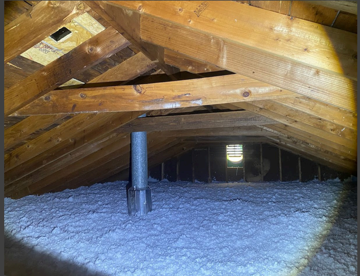
Combustion Flue
